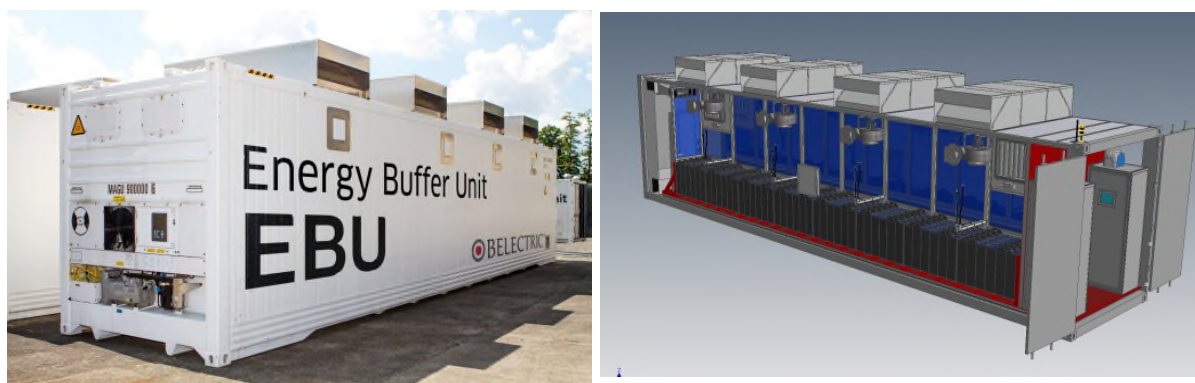
Image 5 (courtesy of Belectric): Energy Buffer Unit (EBU) battery storage
