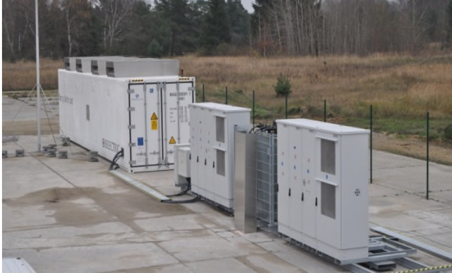
Image 6 (courtesy of Belectric): EBU (battery storage) with inverter installation at Alt Daber, Germany
