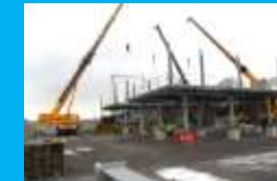
Series Compensation Moffat Platform Erection
