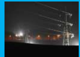
Re-conductoring OHL over M74
