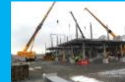
Series Compensation Moffat Platform Erection
