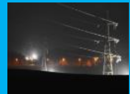
Re-conductoring OHL over M74
