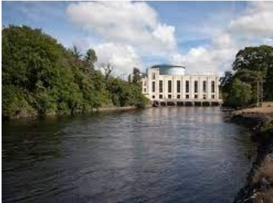
Energised up to 275kV from 11kV 13MVA Generator & measure BLPU of Hydro
