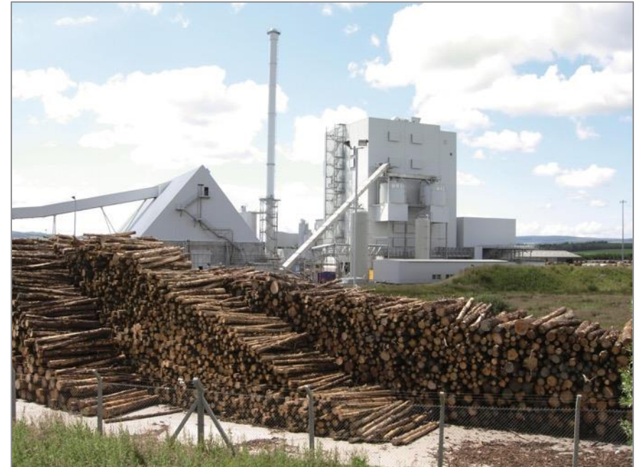
Energised up to 400kV from 33kV 53MVA Generator & measure BLPU of Biomass
