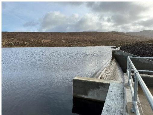
Figure 2 – intake to penstock from Reservoir
