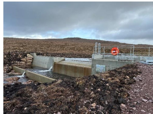
Figure 2 – intake to penstock from Reservoir
